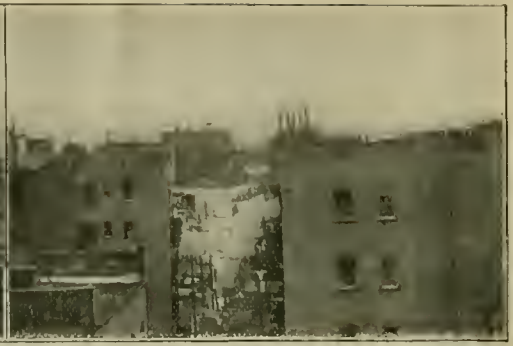
Fig. 10. "WASH OUT ON LINE."
